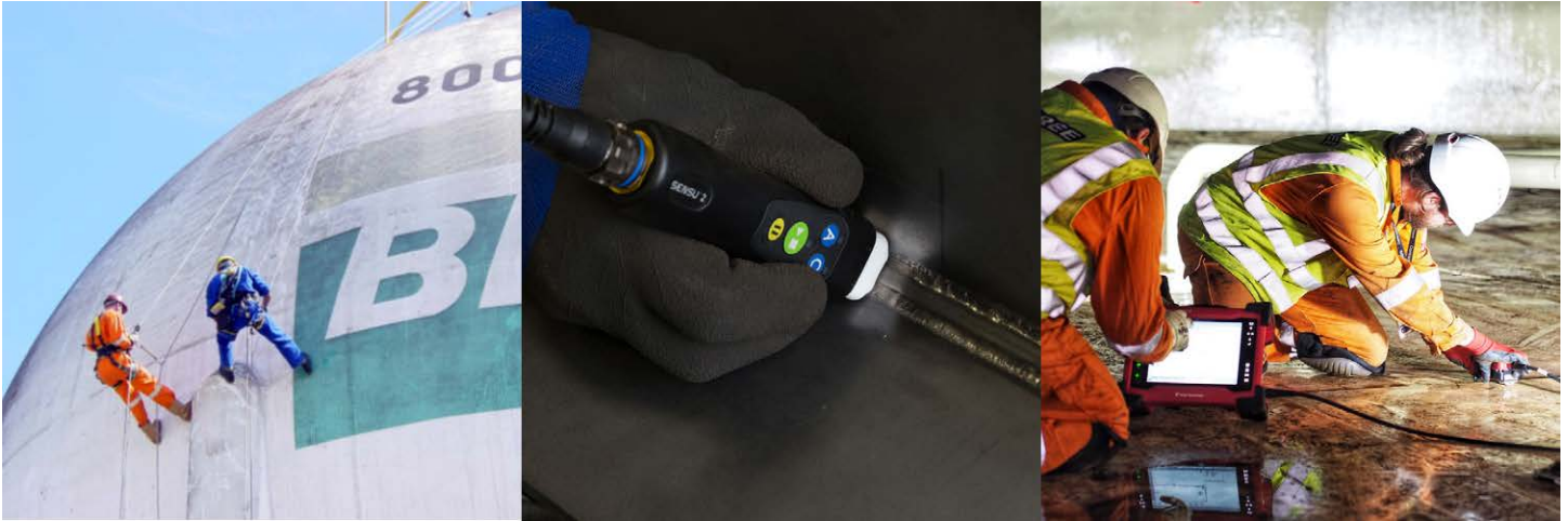
Left to right: Gas sphere inspection, fillet weld inspection, tank floor weld inspection
