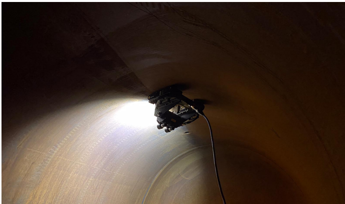
Internal vessel inspection
