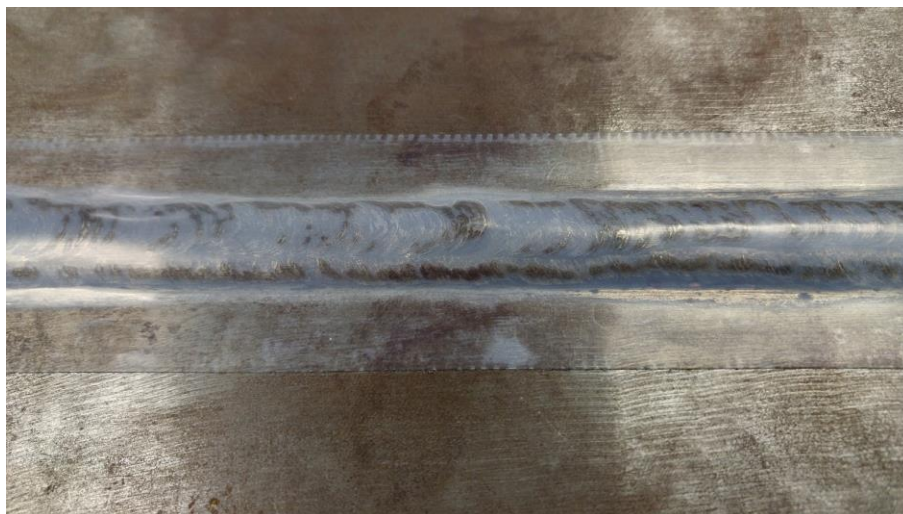
Figure 27. Protective tape applied directly on weld
