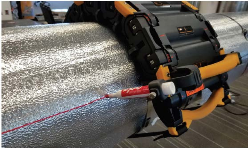
Figure D-9 Installed Grid-As-U-Go
